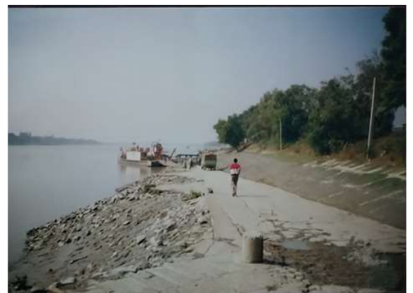
Hasnabad Slipway cum Vehicular Jetty
