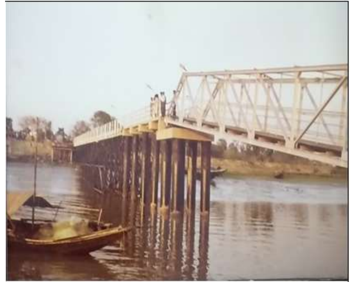
Roychak Jetty in progress
