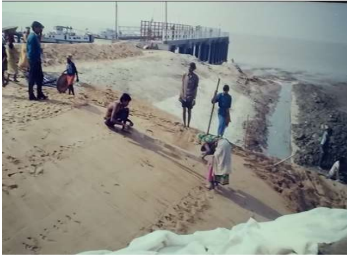
Shore Protection Works using Geotextile in progress
